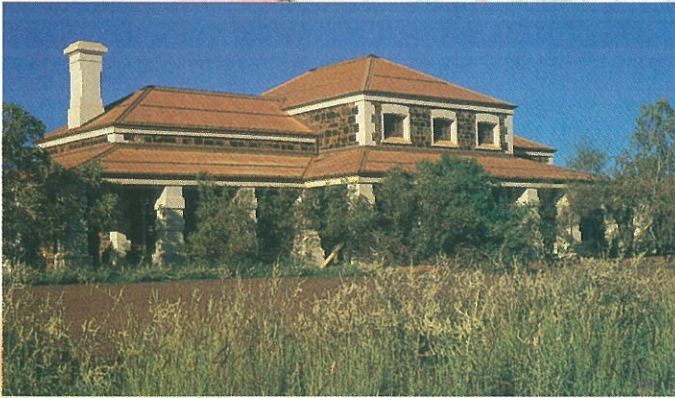
Built of local stone, the Courthouse in Cossack is a monument to the Pilbara's past.
