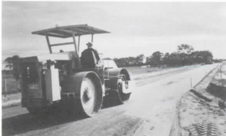
Work on the project.
