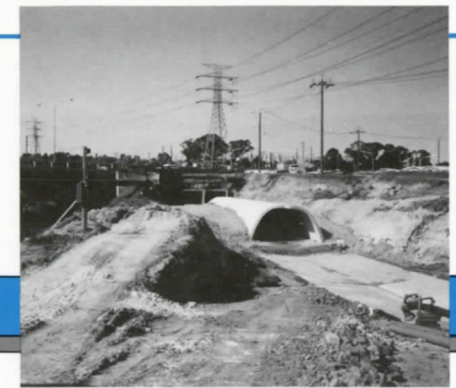
Undergrounding of Scotchmans Creek near Warrigal Road, Chadstone
