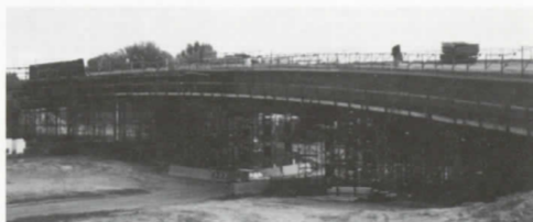
Moira Street/Dunlop Street bridge under construction at Malvern East
