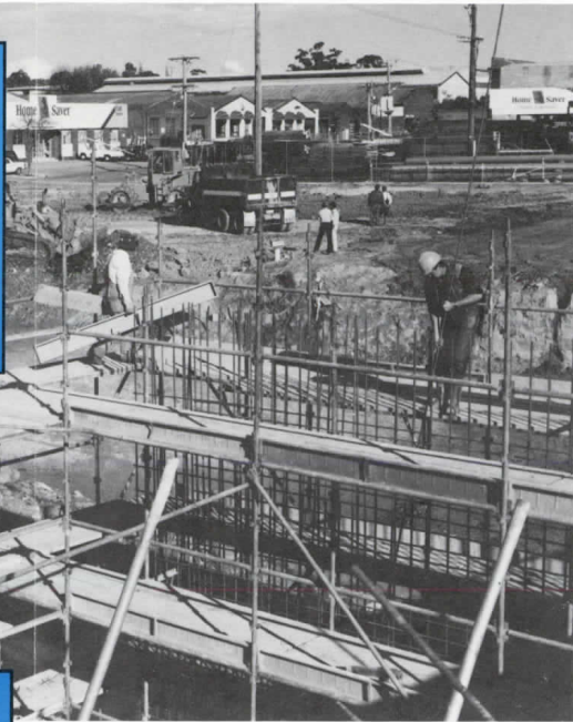
Bridgework on the project
