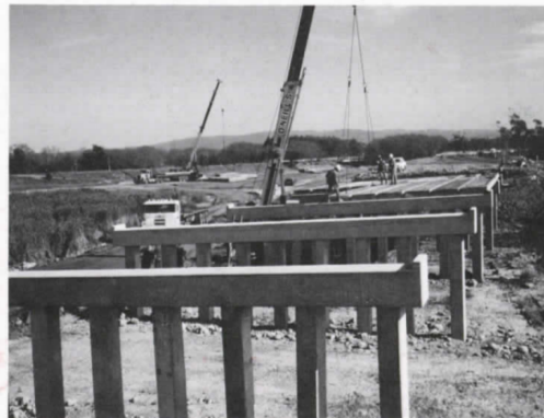
Above: bridgework on the project
