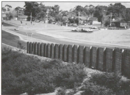
• Noise barriers on Stage 2
