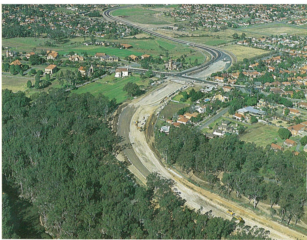
Aerial view of the construction of the North Parramatta By-Pass.
