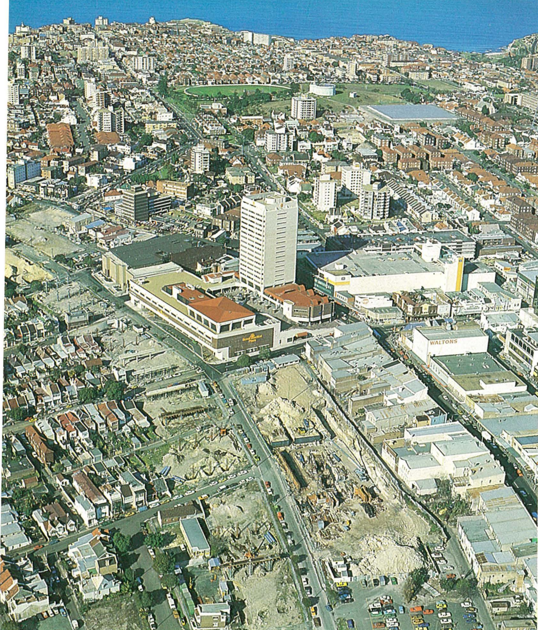
Bondi Junction By-Pass to fit in with the bus-rail terminal under construction at Bondi Junction.
