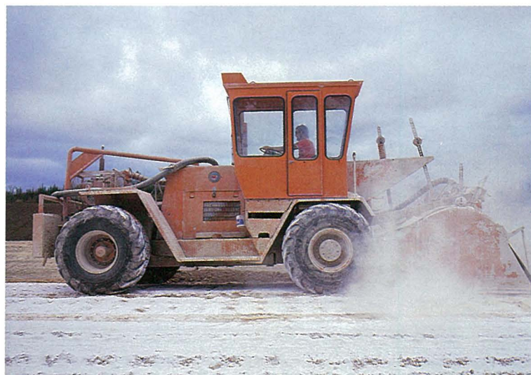
A hopper spreading quick lime (above) as part of the pavement stabilisation process which included mixing and watering (below)
