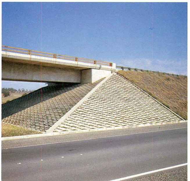
Campbelltown onloading ramp
