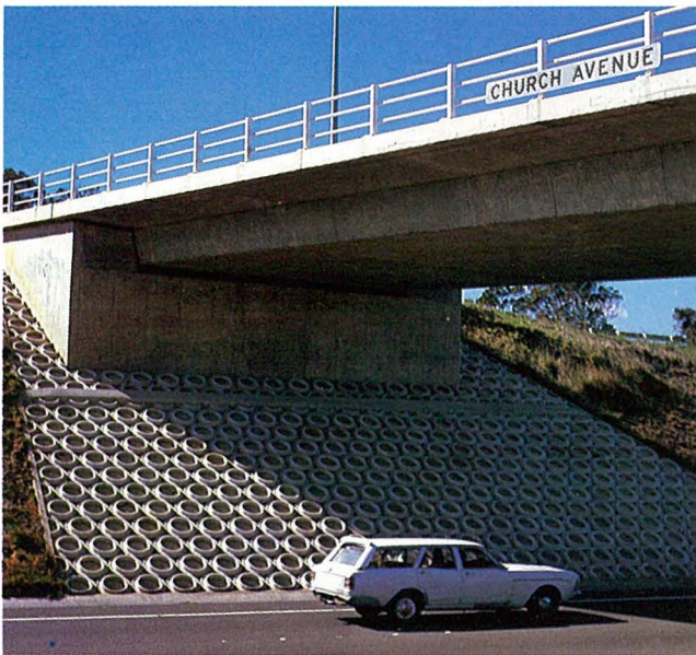
Church Avenue overbridge
