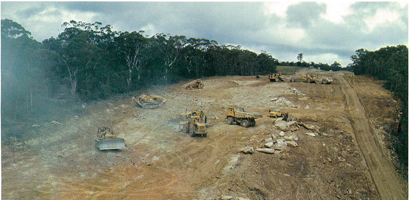
Early stages of earthworks in progress, April 1974.
