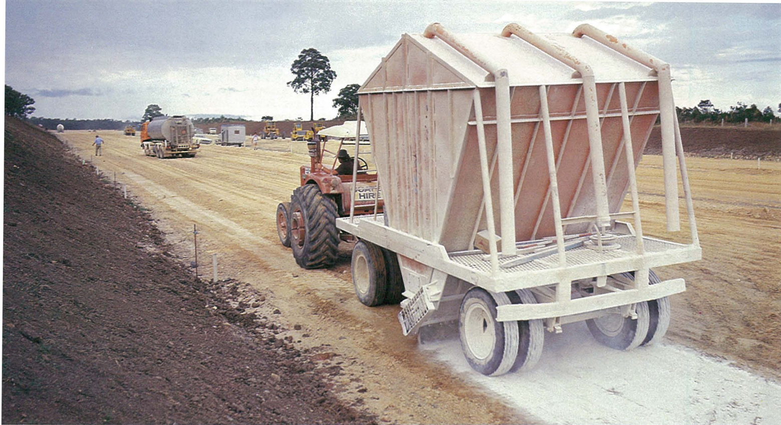
A hopper spreading quick lime (above) as part of the pavement stabilisation process which included mixing and watering (below)
