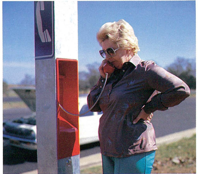
High-technology emergency telephones are situated approximately 1½ km apart along the freeway.
