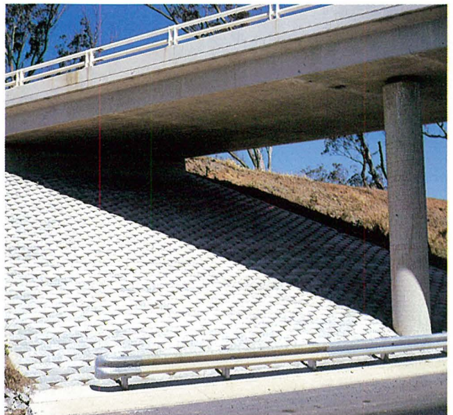
Menangle Road overbridge
