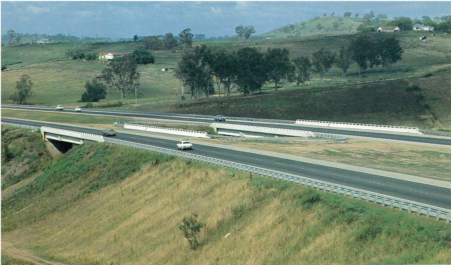
Twin bridge structures carry the South Western Freeway over Aero Road near Ingleburn.
