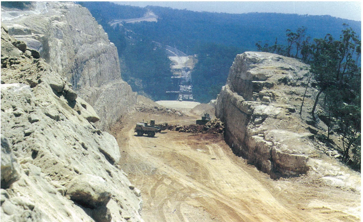
The deepest cutting (40 m) on the project is just east of Mooney Mooney Creek.
