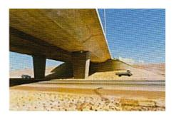
The second crossing over the Tonkin Highway was a 70-metre-long, two-equal-span bridge at a moderate skew of 17 degrees. The overall deck width of 26 metres was achieved by an in-situ, dual-spine, multi-cell, partially prestressed concrete box girder constructed in two stages. Each four-cell girder is connected to the other by a reinforced concrete top
